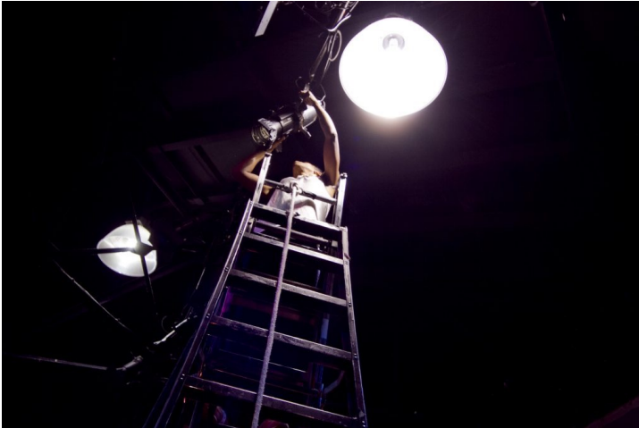
Focusing by hand from ladder very difficult to maintain 3 points of contact
